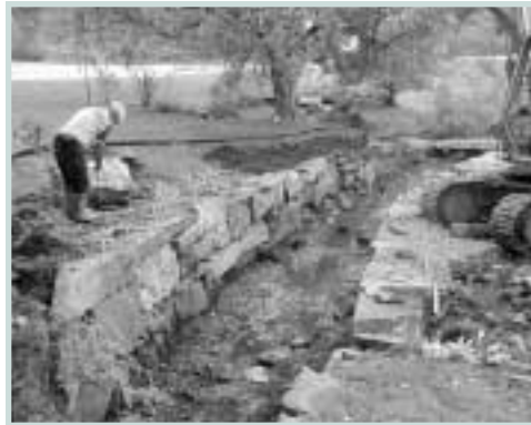
Summer 2001 construction. Rebuilding rock retaining walls and patching lower dam. Look for more construction photos continued throughout the newsletter. — All construction photos taken by Eric Ryea
