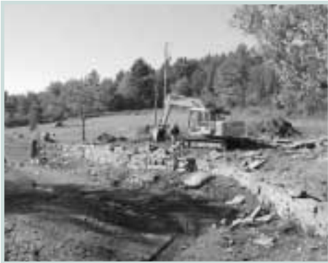
Summer 2001 construction. Rebuilding rock retaining walls and patching lower dam. Look for more construction photos continued throughout the newsletter. — All construction photos taken by Eric Ryea
