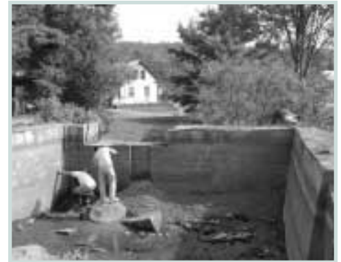
Summer 2001 construction. Rebuilding rock retaining walls and patching lower dam. Look for more construction photos continued throughout the newsletter. — All construction photos taken by Eric Ryea
